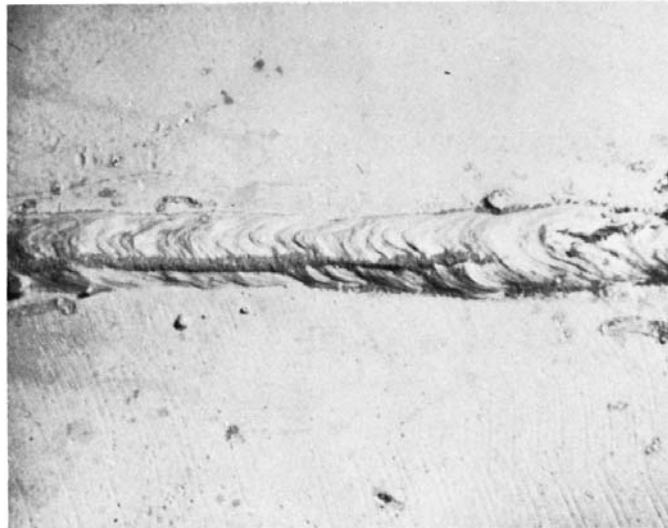
FIG. A1.20 Indication of Surface Cracks (Produced by Prod Magnetization, AC Continuous)
